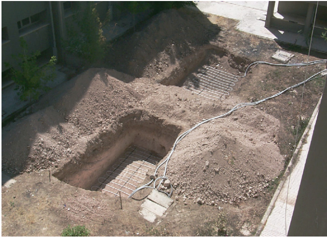
Fig. 2. The view of the ground heat exchangers buried at 1 and 2 m depths.
